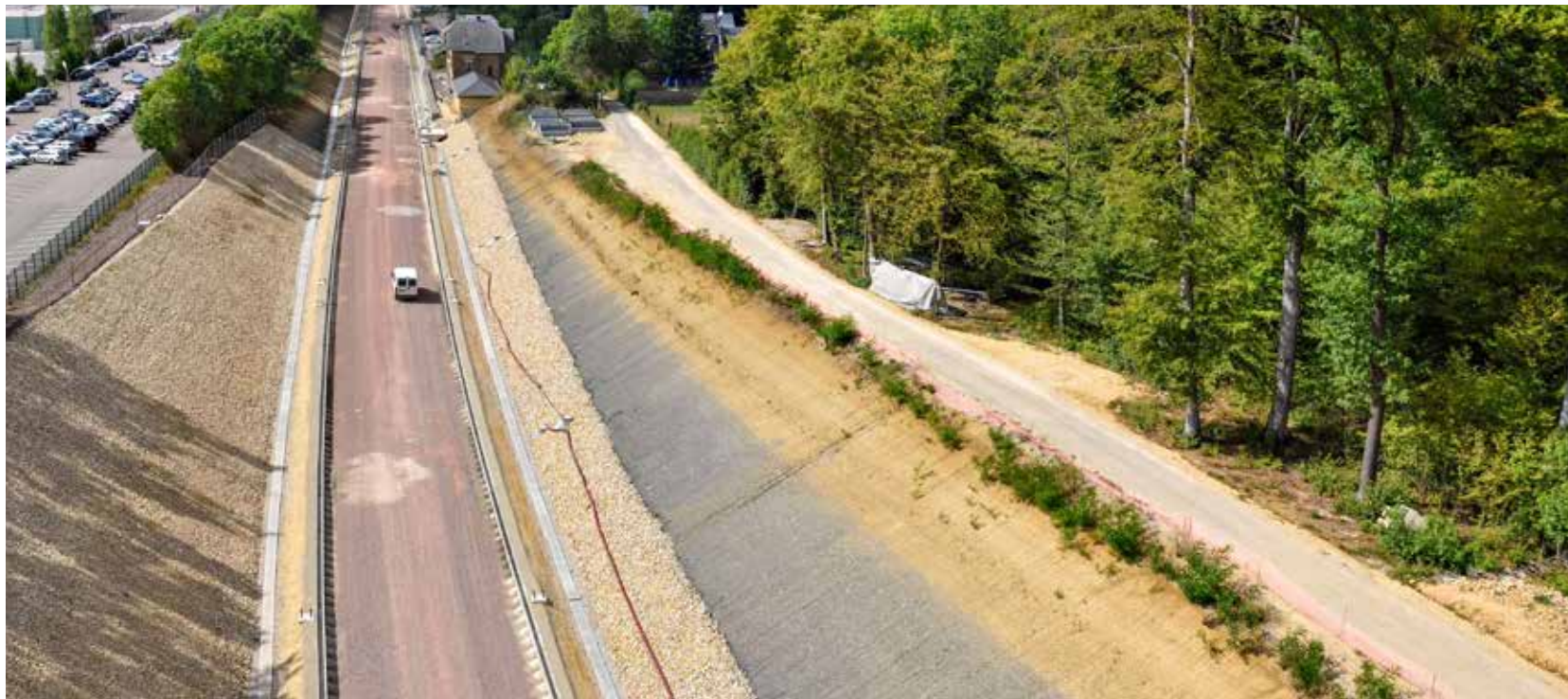
SECOND TRACK ON LUXEMBOURG-SANDWEILER RAILWAY
