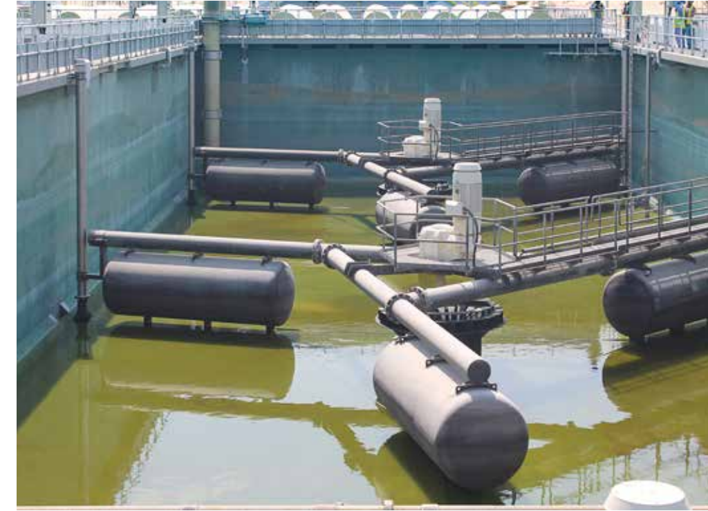
AL SAJA'A TANKER DISCHARGE FACILITY & SEWAGE TREATMENT WORKS Sharjah, UAE
